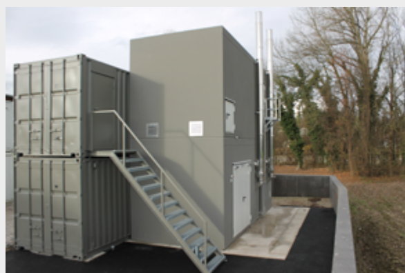
Doppelstock-Heizcontainer 2x90 kW Pellets, Industrie
